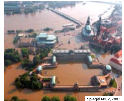
Spiegel No. 7, 2003 Figure 1: Flooding of the city of Dresden in 2002.
